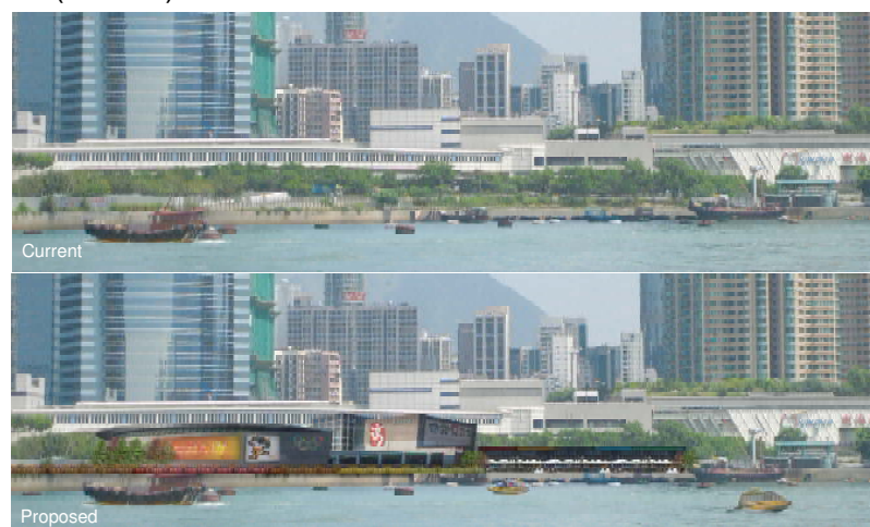
Photomontage showing the waterfront node at the northern edge of the Yau Ma Tei Typhoon Shelter.
