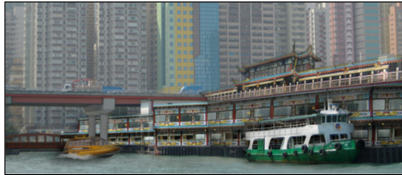
Photomontage showing renovated North Point (West) Ferry Pier
